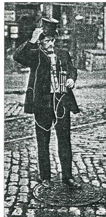
Manhole as a ground
